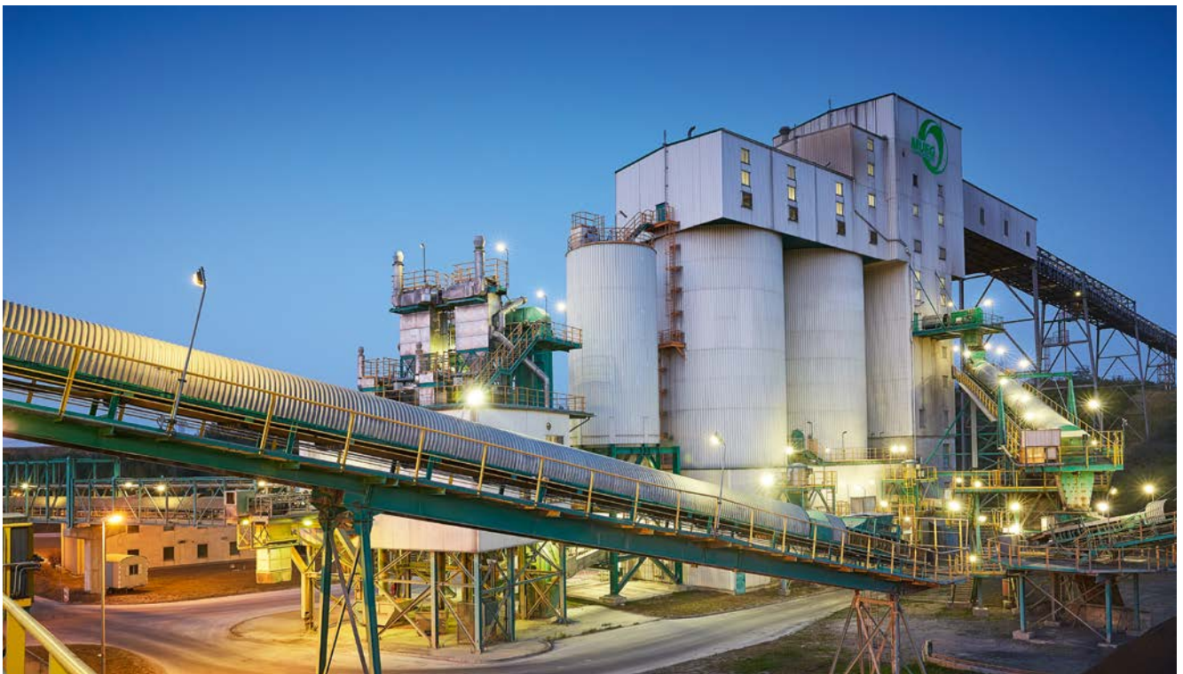
Peres recycling plant, serving Lippendorf power plant
